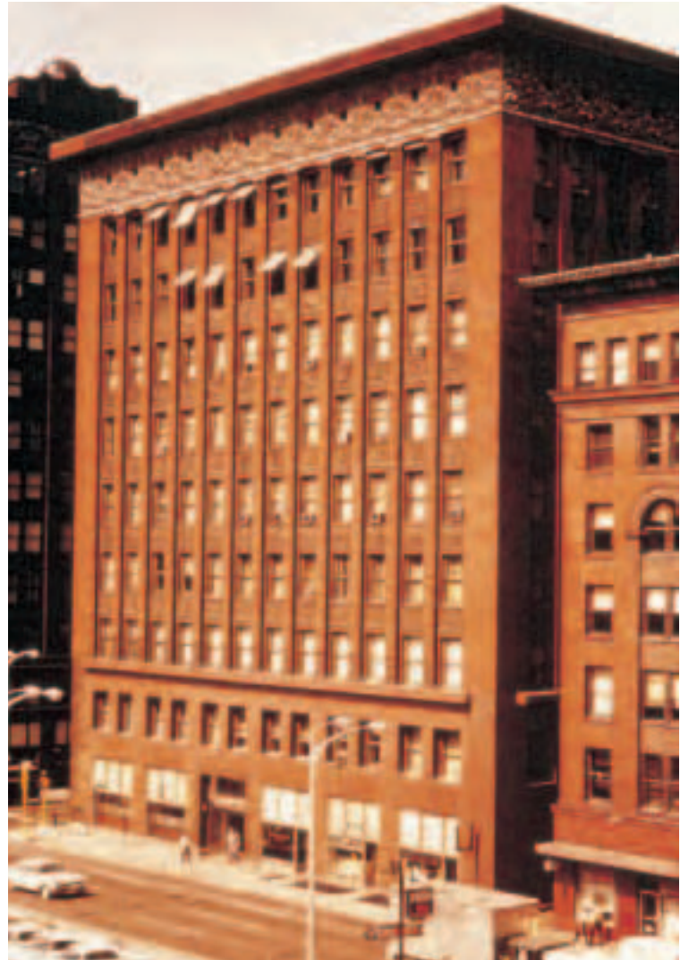
► FIGURE 3.17 This skyscraper echoes its internal steel frame in its exterior design. Sullivan emphasized the height of the skyscraper by stressing the vertical lines that move the viewer's eyes upward, and underplaying the horizontal elements in the window area.
