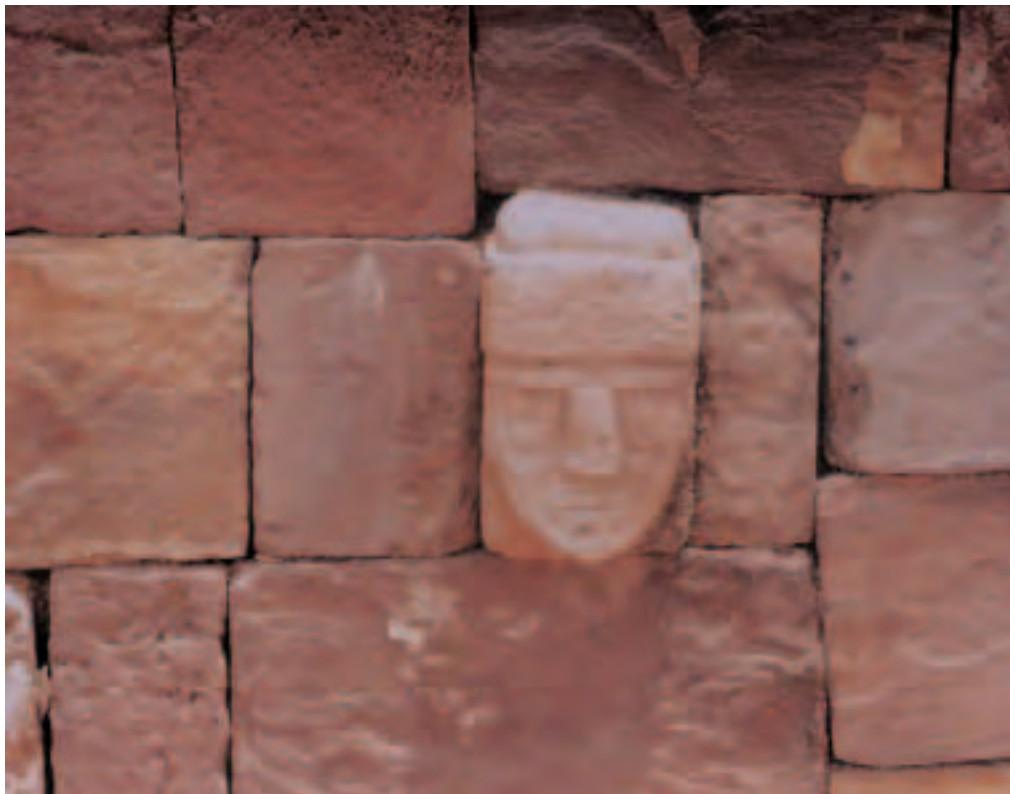
◀ FIGURE 3.16 The builders of Tiwanaku in present-day Bolivia were excellent stone masons. They cut the stones to fit together so perfectly that the buildings have survived to this day without any mortar to hold the stones in place.
